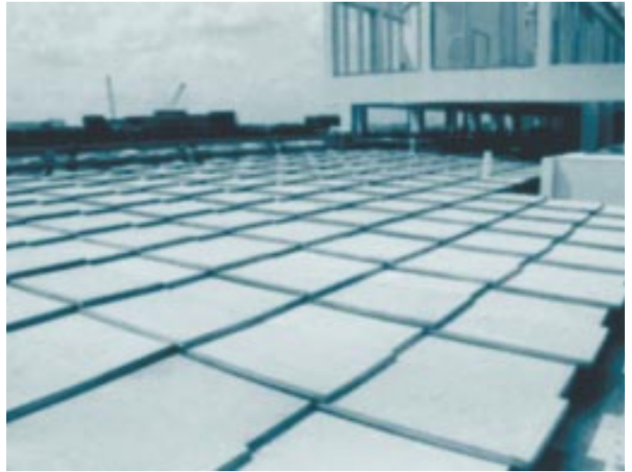
This is one of the trial installations in Sembawang.
